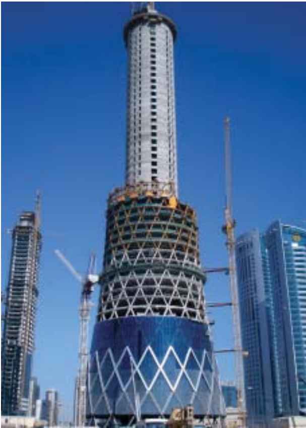
Qipco Tower, one of Eversendai's projects in the Middle East.
